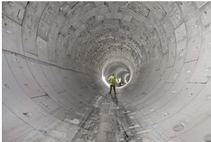
Fig.1.1. Tunnel linings in London metro built from precast FRC panels
