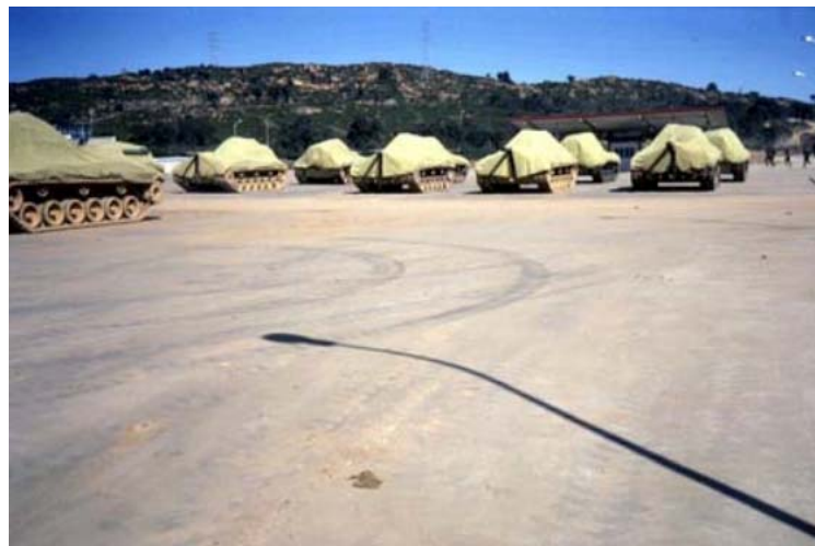
Fig.1.4. FRC Pavement in Cordoba (Spain). Figure from [20]
