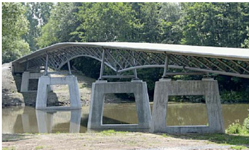
Fig.1.5. Pedestrian bridge in Kassel (Germany) built from HPFRC supported on a 3-D steel truss
