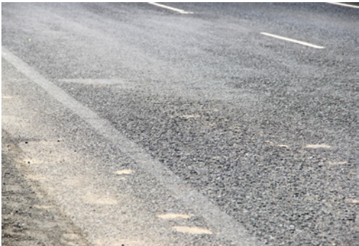
Figure 2. Ravelling on pavement section NH-8GJ at 434.00 km
