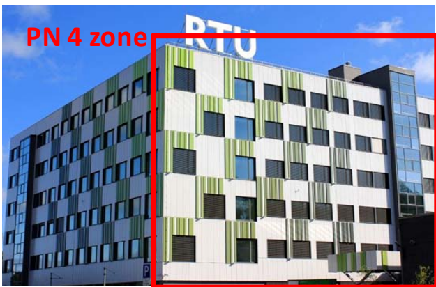
Fig. 1. Faculty building south facade and PN4 zone.
