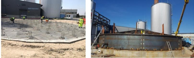
Fig. 4.1. Basic arsenal works of heat accumulator and assembly of metal structures (author's photo).
