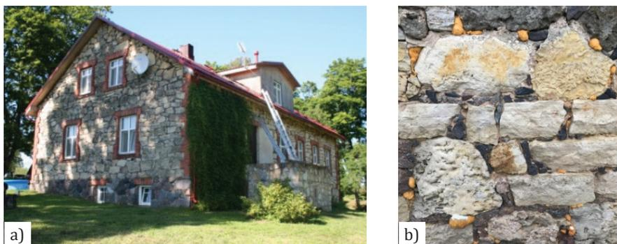
Fig.1.6. Historical building of dolomite stones in Seces parish: a) the main facade of the building; b) the outer surface of the stone wall.
