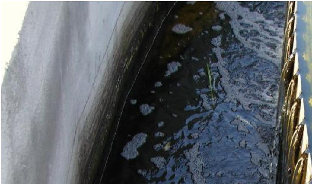
Figure 4.13. Effluents launder with overflow weir
