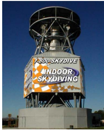
Fig. 6. The aerodynamic stand with open circuit and closed working section Sky Venture "(USA, Florida).
