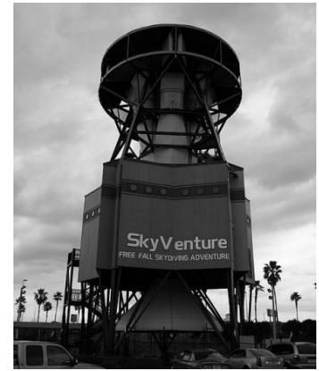
Fig. 6. The aerodynamic stand with open circuit and closed working section Sky Venture "(USA, Florida).
