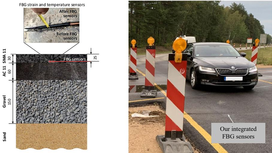
Fig. 3.2. Embedded FBG sensors on the carriageway in locations (a) and (b).
