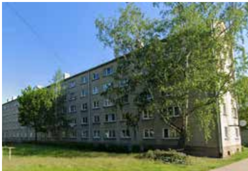
Figure 38. A five-storey residential building of the 1-430 series standard project in Riga, 30 Patversmes Street (GoogleMaps).
