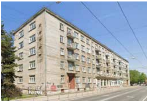
Figure 39. A five-storey residential building with a shop of the 1-430 series standard project in Riga, at the intersection of Valdemāra and Zirņu Streets (GoogleMaps).
