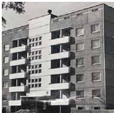
Figure 102. Five-storey experimental building of the 119 series standard project in Iļģuciems, on V. Tereškovas (now Bulļļu) Street (1970s).
