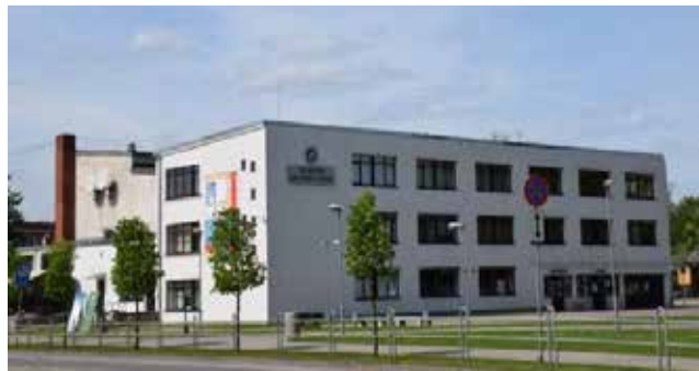
Figure 93. Valmiera Culture House, built according to standard project L2-06-08 (2020).
