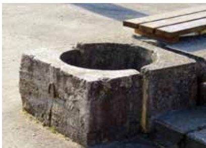
Figure 109. Prefabricated reinforced concrete waste bins in Ķīpsala (2008).
