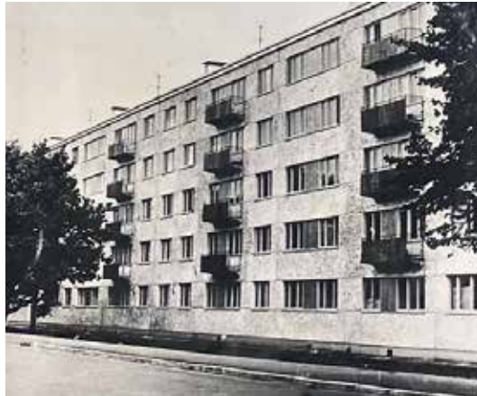
Figure 73. The first five-storey residential building of the 467 series standard project in Riga (residential complex on Raunas and Bīķernieku Streets, 1970s).
