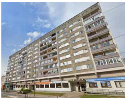
Figure 75. A nine-storey residential building of the 1-467 AL-68/2 series standard project in Riga, Maskavas Street (GoogleMaps).
