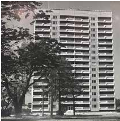
Figure 83. A twelve-storey residential building of the 104 series standard project with six apartments on each floor and a loggia in the living room in Riga, Ogres Street (sections 1-1-2-2-3-3; 1970s).
