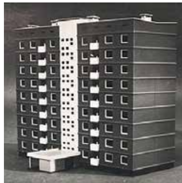
Figure 101. Model of a nine-storey experimental building of the 119 series standard project (1970s).
