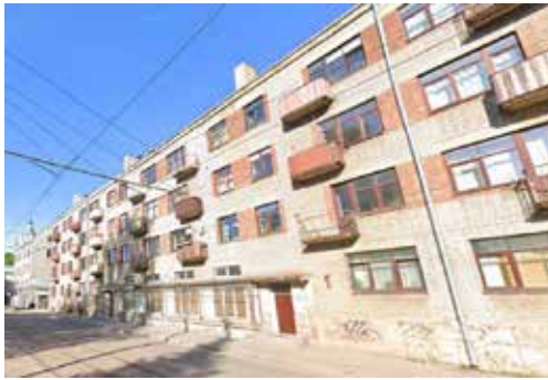
Figure 36. A four-storey residential building with a shop of the 1-430 series standard project, in Riga, 76 Slokas Street (GoogleMaps).
