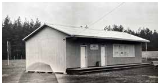
Figure 62. A 2-2-2 section two-room apartment module of the 1-316 series standard project at the Construction Exhibition in Mežaparks (1957).
