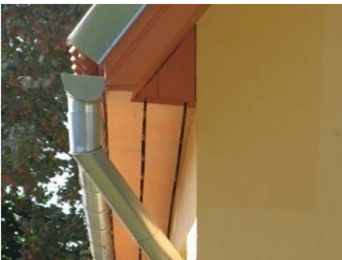
Fig. 9 and 10. On the left – insulated building, where instead of cornice is constructed “wind box”. On the right – cornice with jagged band peculiar to Kuldīga old town. Buildings can be insulated only from inside not to lose cornice solutions and brick elements.
